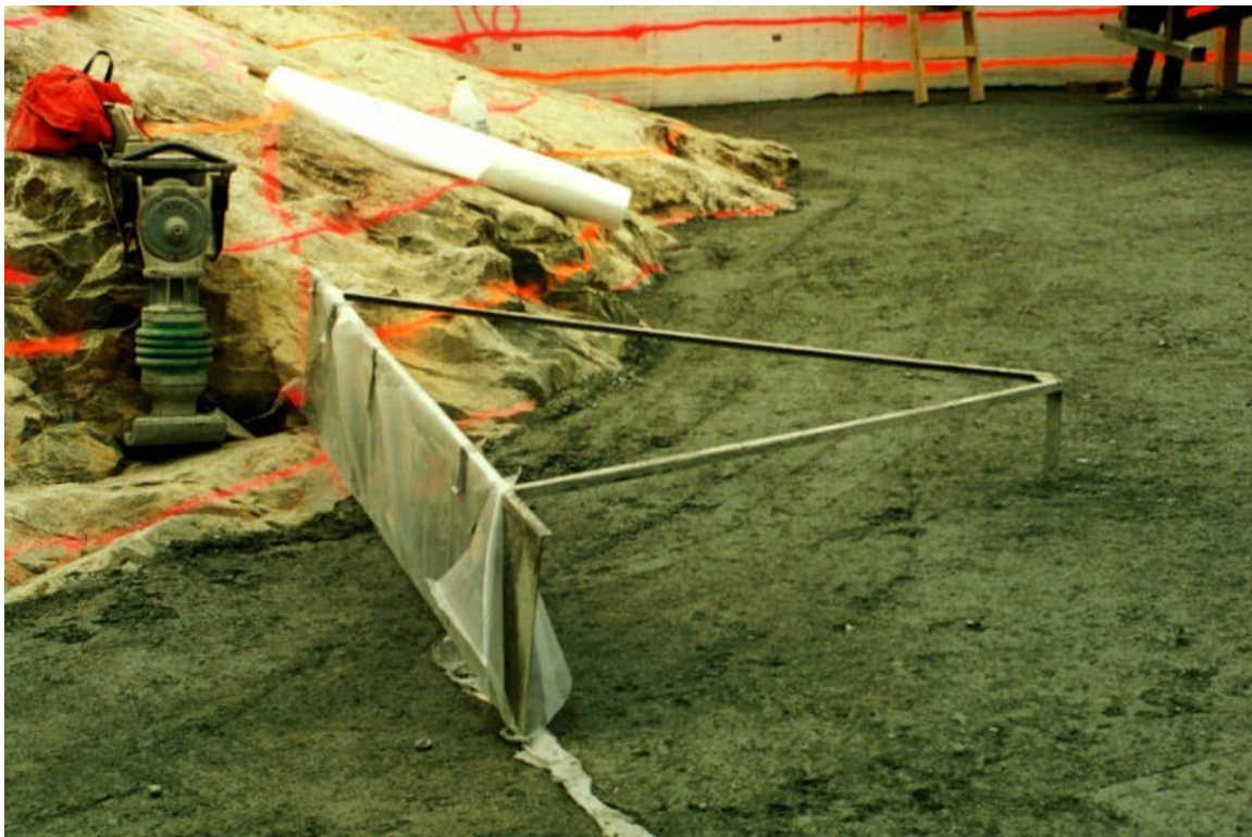
Figure 6-4. Transverse contraction joint construction with plastic-wrapped joint form
